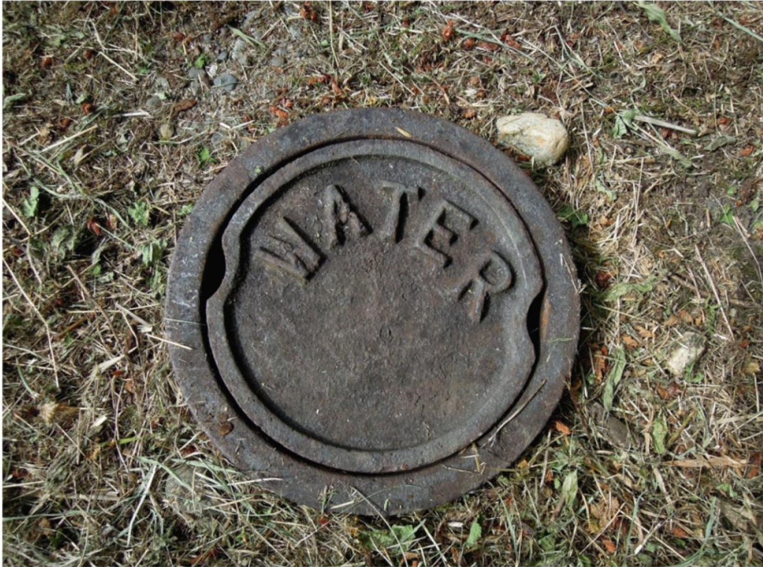
Photo: Nelson valve box Photo credit: Kama Corbett
